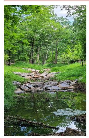
The SWM Pond Retrofit and Stream Restoration projects in Montgomery County entailed the retrofitting of the existing Flint's Grove Stormwater Management Pond and the restoration of approximately 1,200 linear feet of stream.
